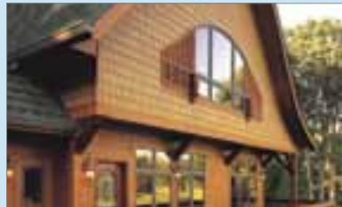
Fiber Cement Siding
